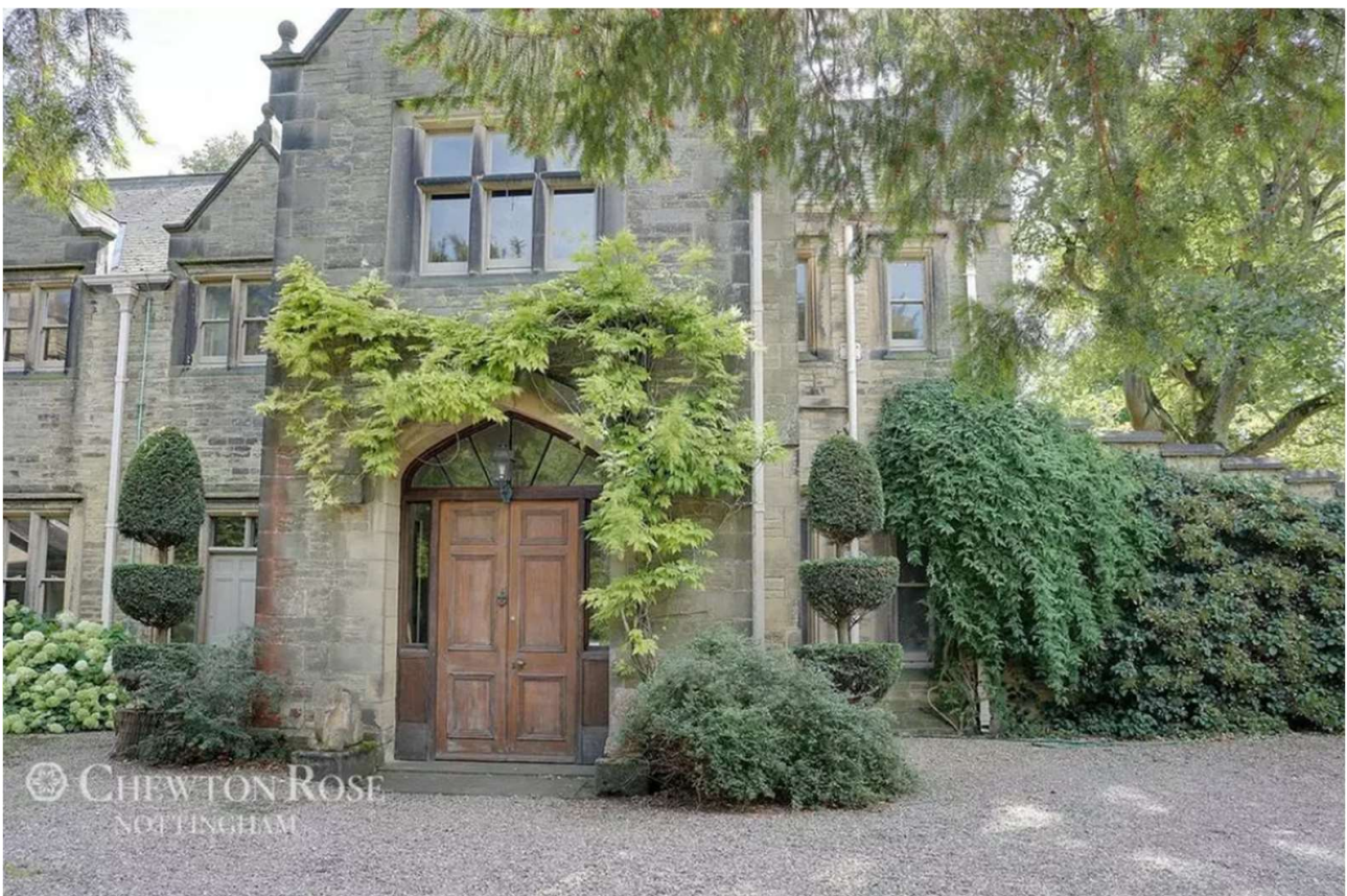
Figure 2: The original Manor building and main entrance to Teversal Manor
